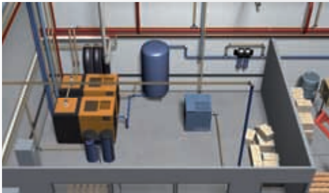
A conventional compressor, with external filtration equipment and high noise operation, has to be placed away from the production area. This lack of integration can raise installation costs.
