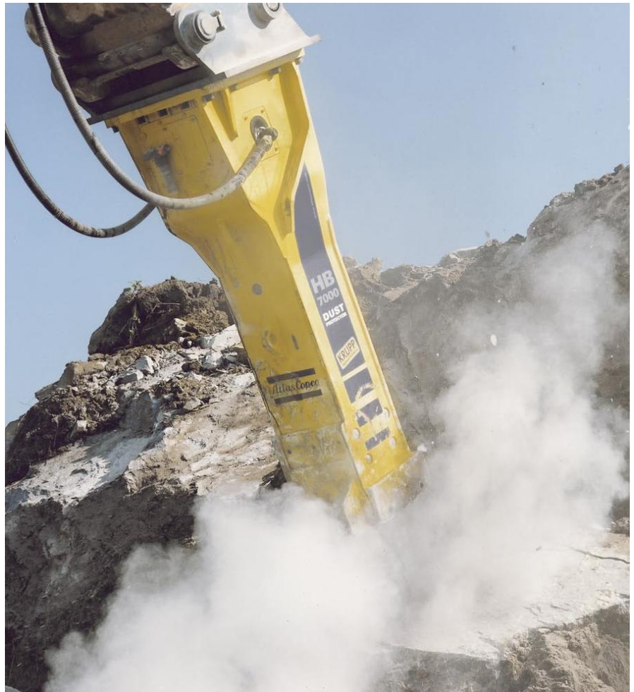
Hydraulic breaker HB 7000 at work.
