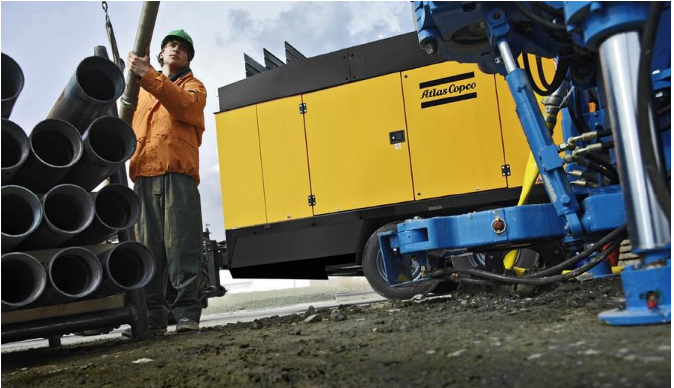
Portable silenced compressor in operation.
