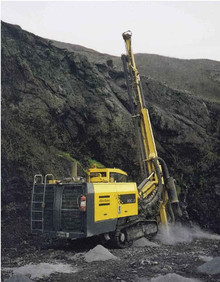
Sleeman ROC L8 bench drilling at 15 degree angle.
