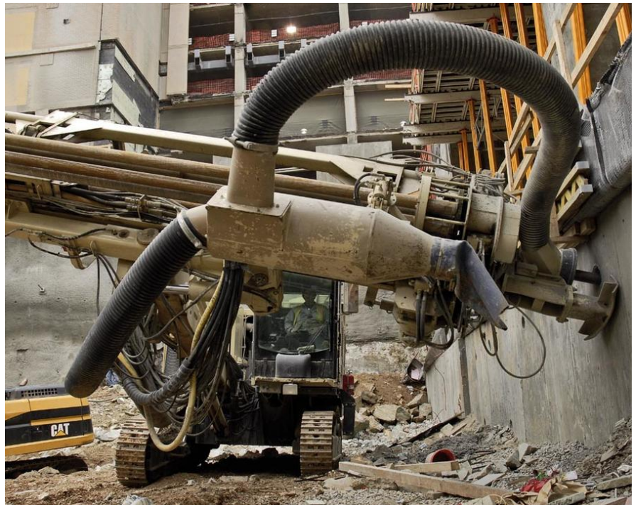
The ECM 780 drilling anchor holes in the excavated wall.
