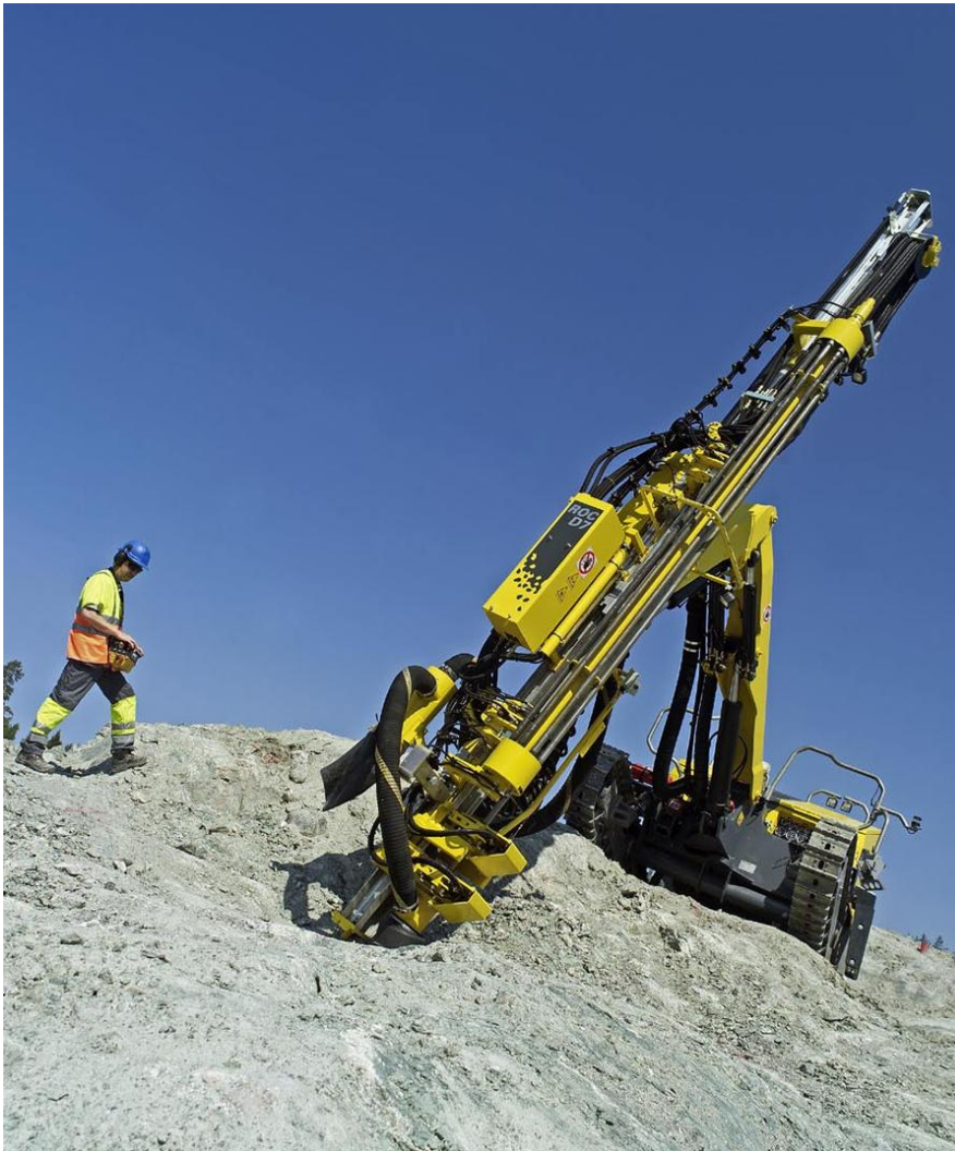
ROC D7RRC with radio remote control offers a safe and effective alternative for difficult and dangerous ground conditions.
