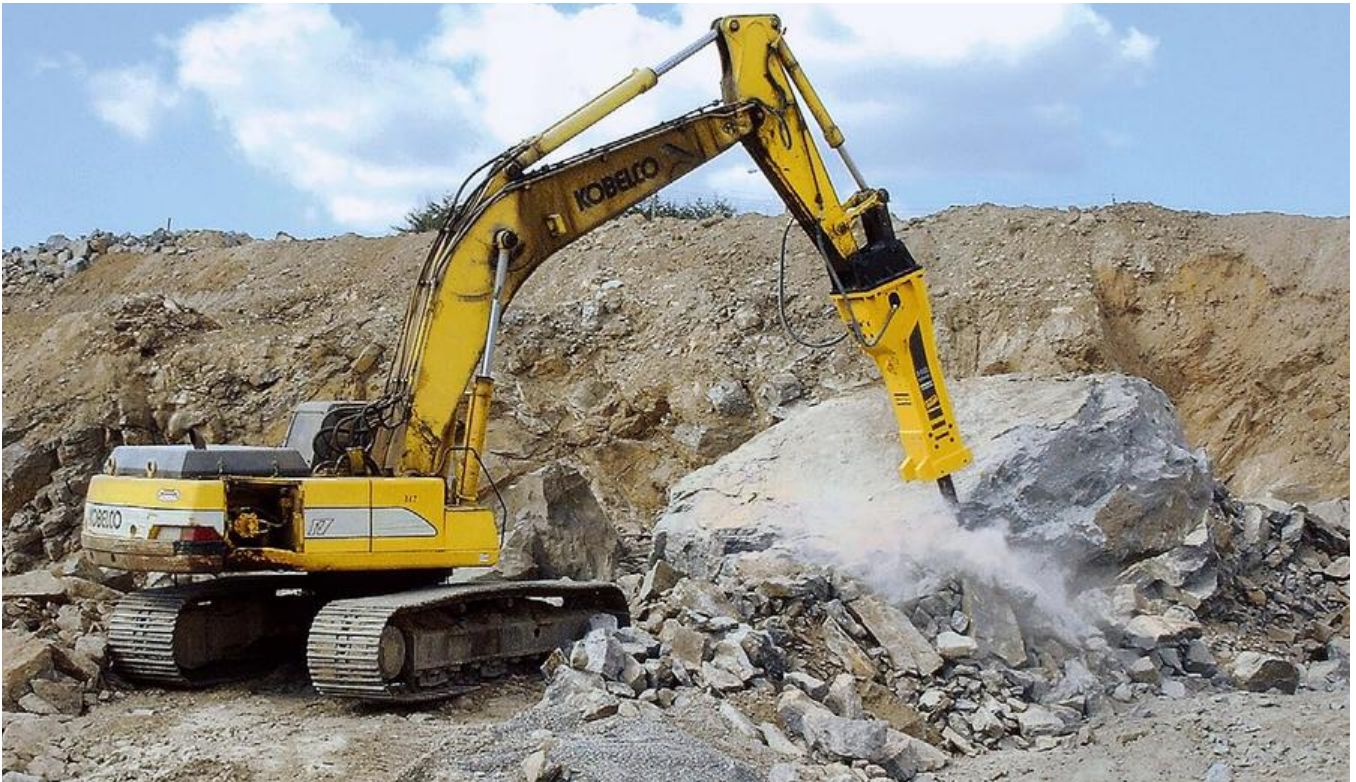
An HB 5800 breaking up a large oversize boulder.
