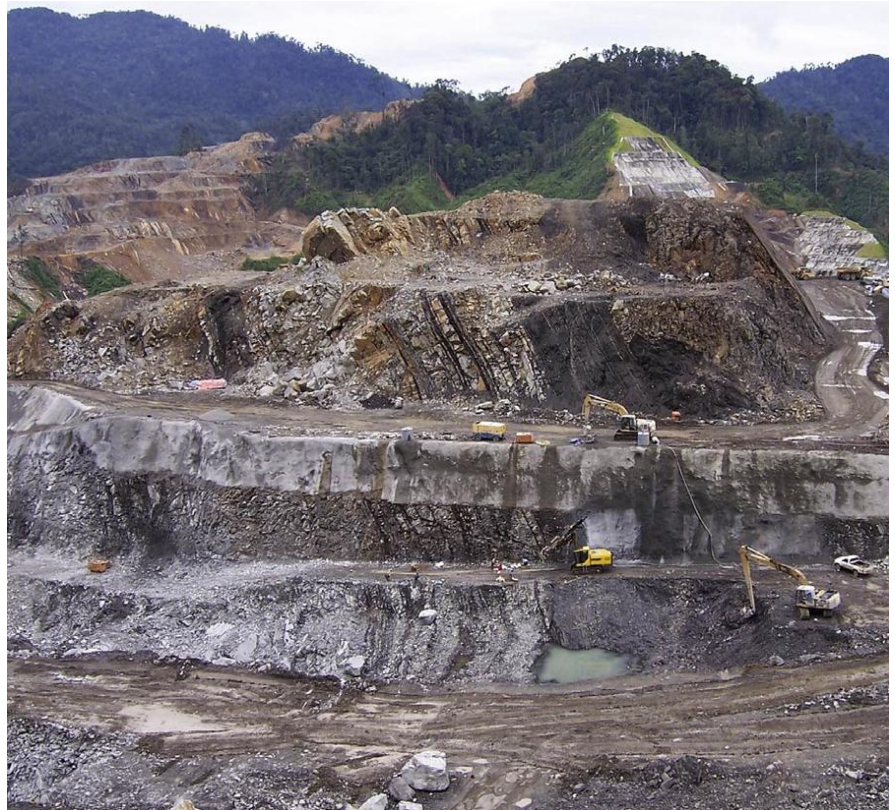
The ROC F7 working on one of the many benches at Bakun.
