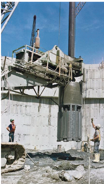
Clusterdrill for construction work
