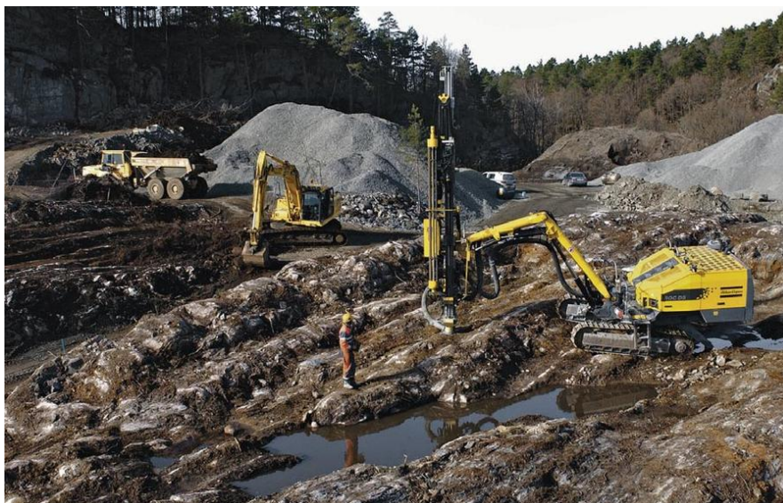
Terrengtransport ROC D7RRC working at Lindesnes, Norway.
