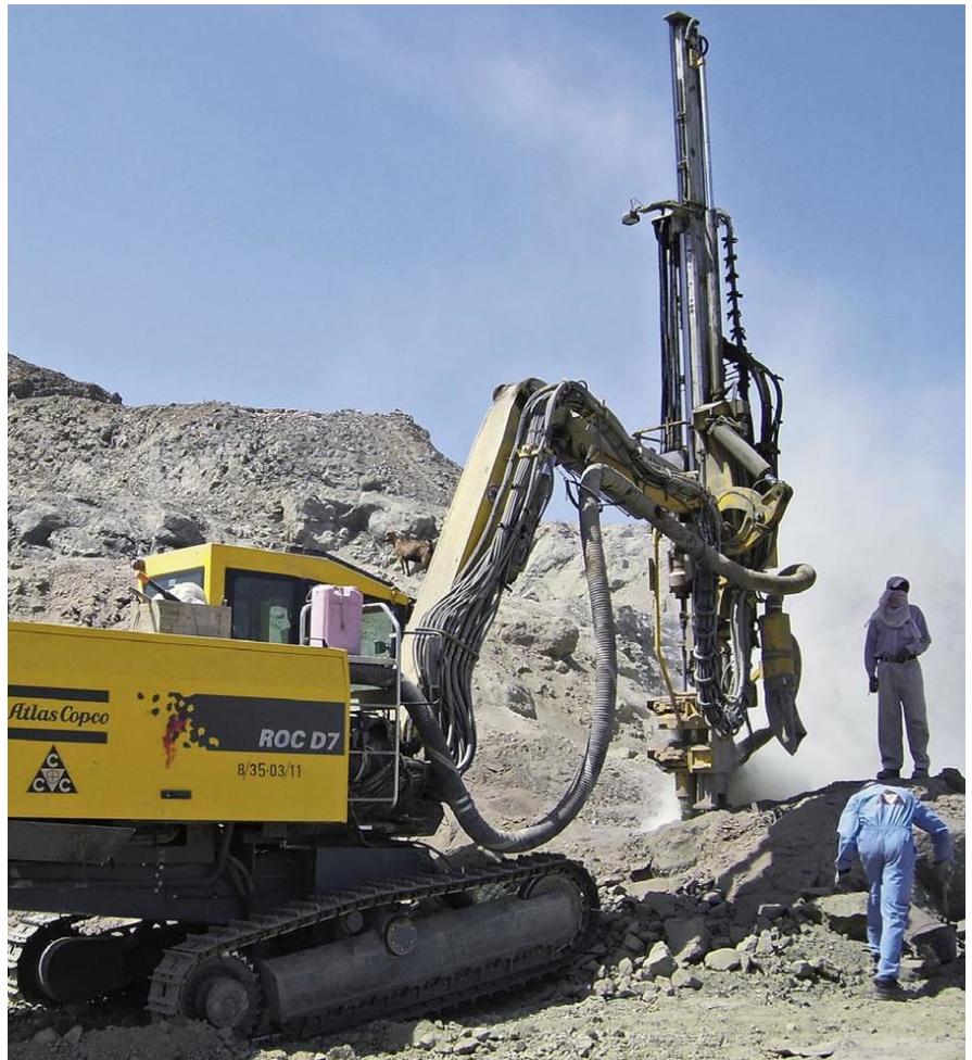
ROC D7 copes well with rough terrain near Muscat.
