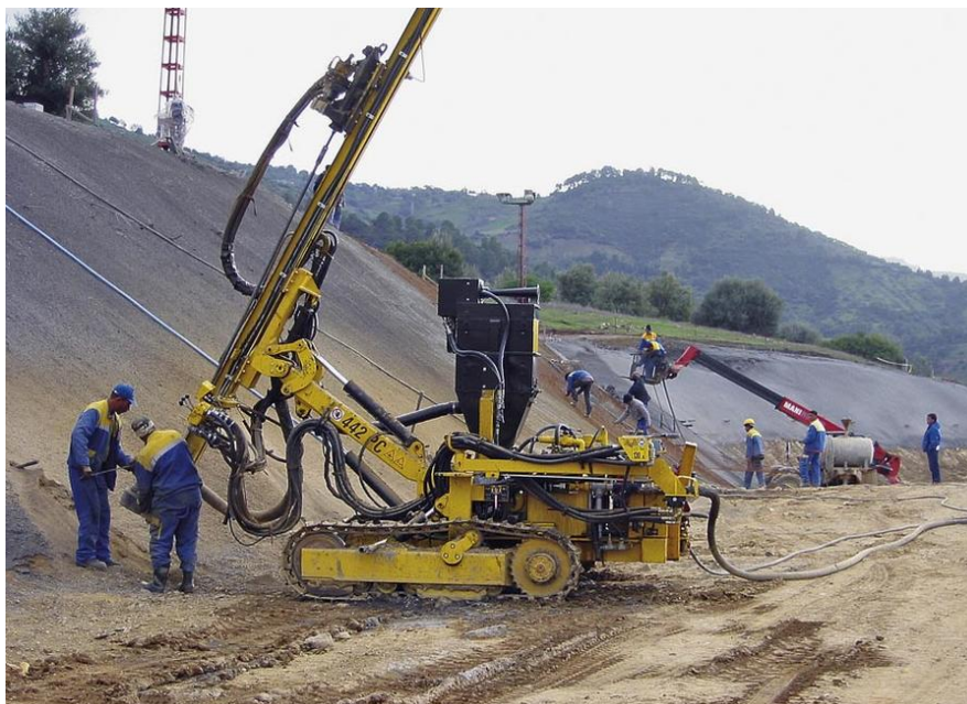
Installation of MAI Self Drilling Anchors with a ROC 442PC and a MAI grout pump m400NT.
