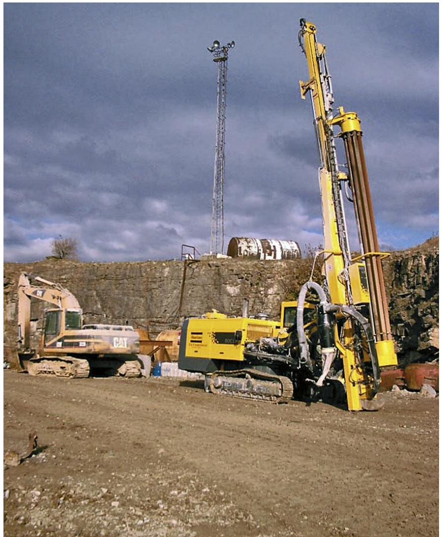
R&B Rockdrillers' ROC L8 moving to new position at Hope Quarry.
