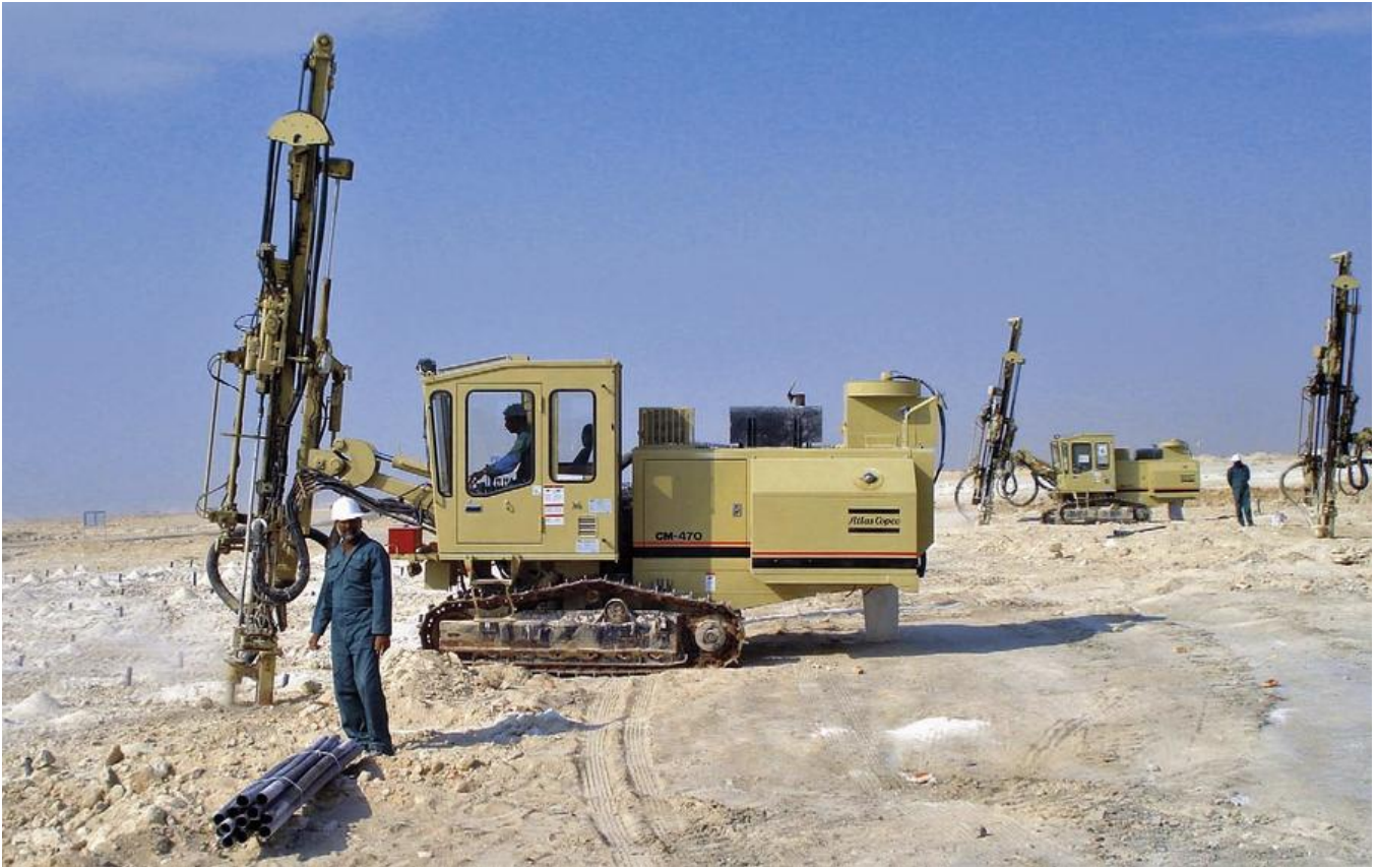
A minimum of 1,200 holes per day: after drilling through the coral limestone, PVC pipes are inserted to keep the holes open for charging.
