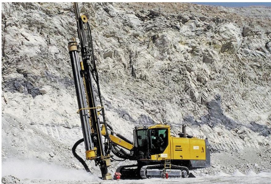
The ROC L8 DTH crawler drill was developed for pre-splitting and large scale production work.
