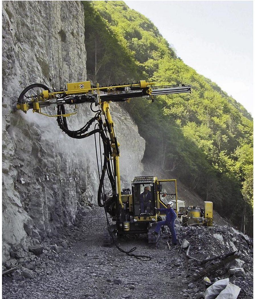
Installation of SDA R38 N with ROC D7 at Carriere d'Arvel, Switzerland.
