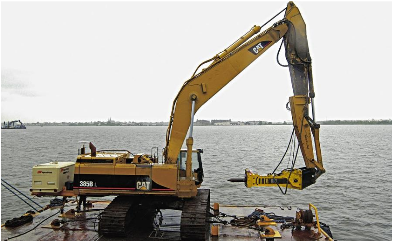
Atlas Copco HB 7000 breaker mounted on CAT excavator at Arthur Kill River.
