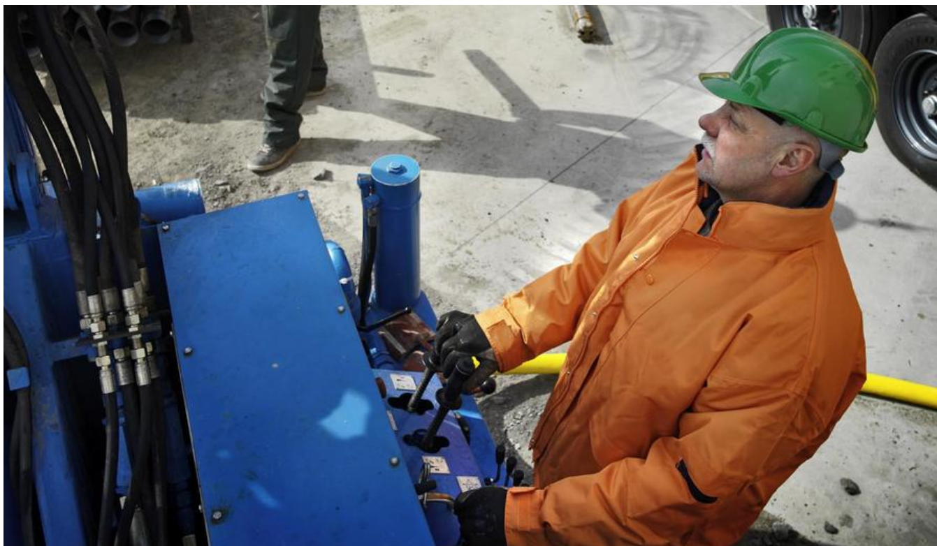
Operating a rig using a towed compressor.
