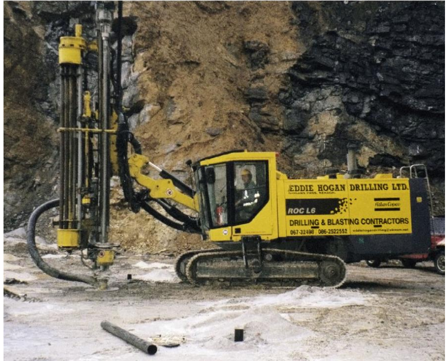
Hogan ROC L6 drilling at Tobin's Quarry, Limerick.
