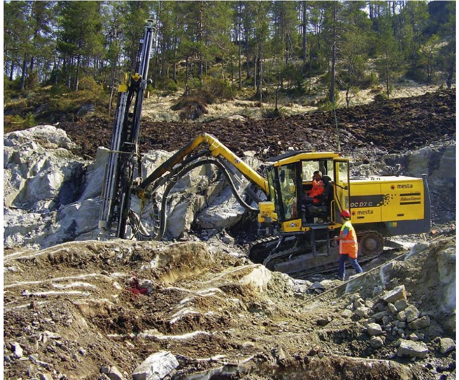
Atlas Copco SmartRig ROC D7C working at Romarheim road improvement project.
