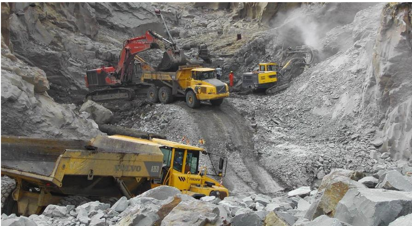
Clearing bedrock for dam foundation.
