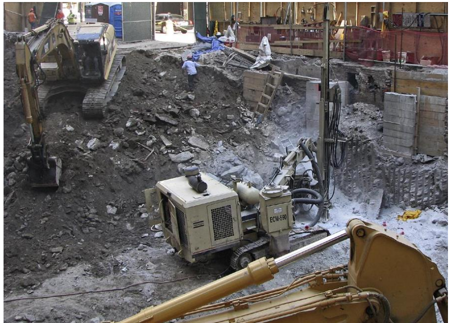
ECM 590 drill rig hard at work in Manhattan.
