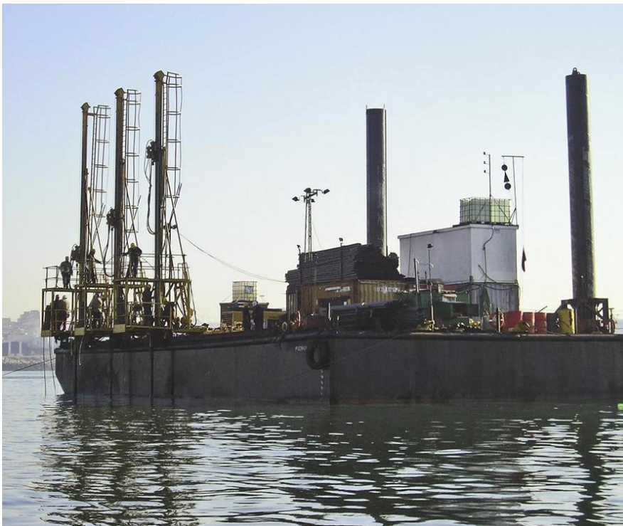
Rockfall barge with three tower rigs mounting BBE 57 pneumatic rock drills.
