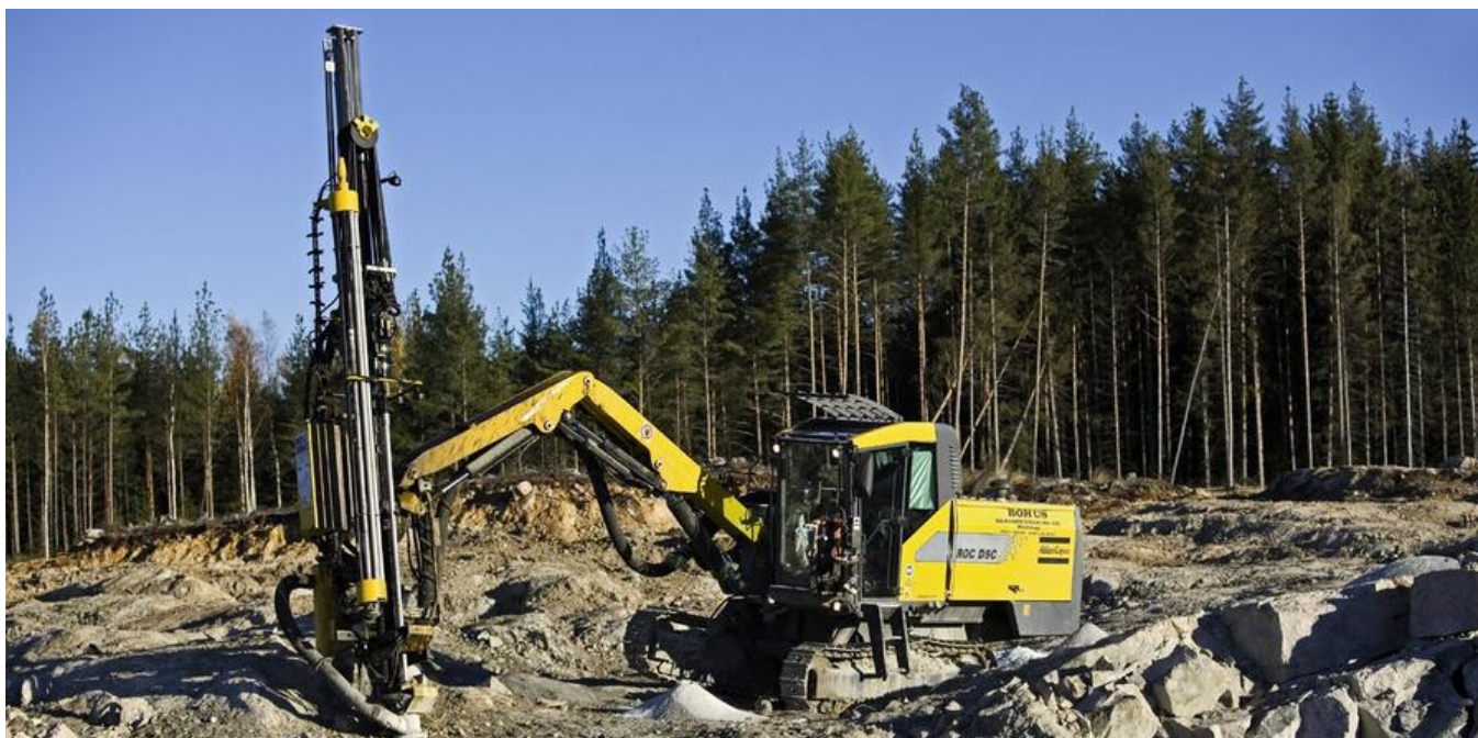
ProCom monitors rig status around the world.
