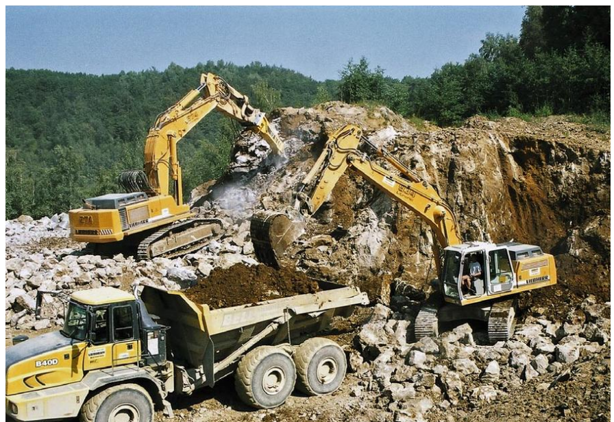
Rock breaking and mucking.
