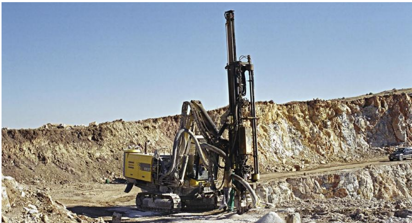
Çektas' old generation ROC D7 has been giving long, high-production service at the Yibitis-Lafarge Lalahan Quarry near Ankara.
