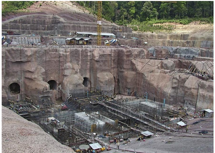
Power house work at Nam Theun 2 dam.
