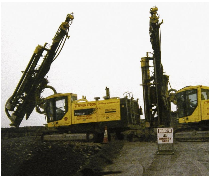
Stephen Lydon operates four ROC F9 rigs with COPROD and two ROC L6 rigs with DTH.
