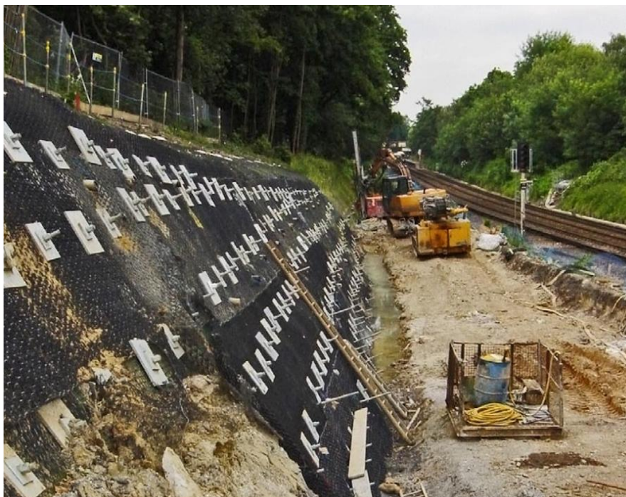
Galvanized MAI-SDA R 25 and R32 anchors installed into loose and collapsing ground using simultaneous drill and grout at the Shortlands Junction, Bromley, Kent, UK.
