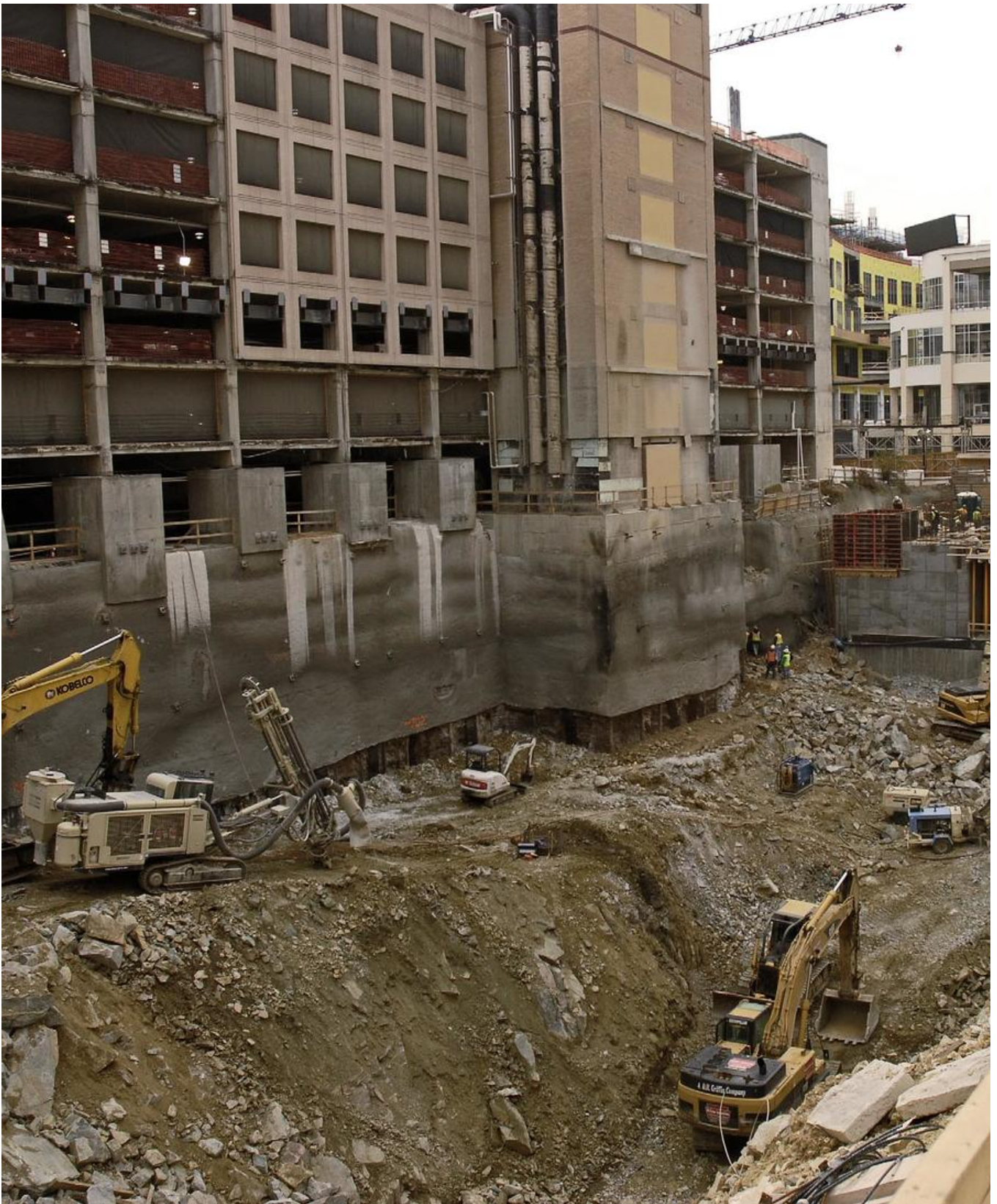
An ECM 780 tramming down the bank after finishing a line of holes.
