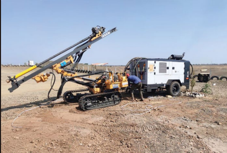
Blast Hole Drilling
