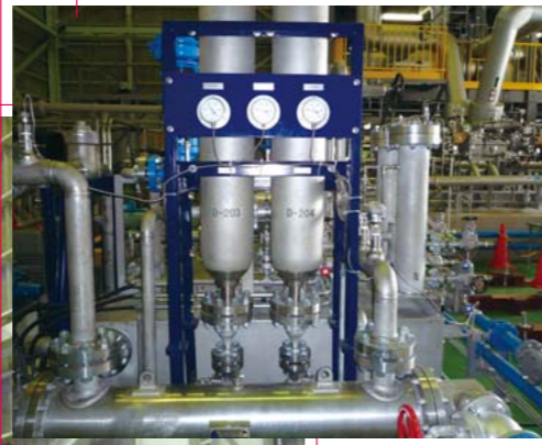
Seal Water Unit for Steam Compressor
